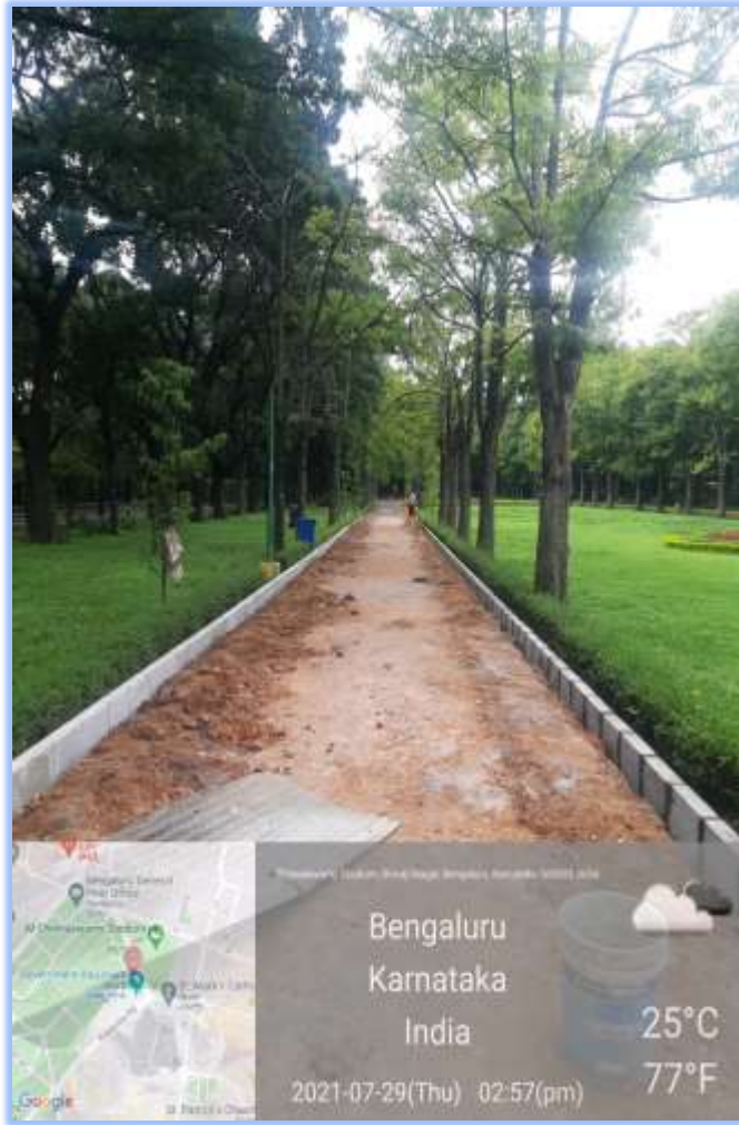
Footpath Improvements, Jogging Track, Laying of Pavers in progress September 2021
