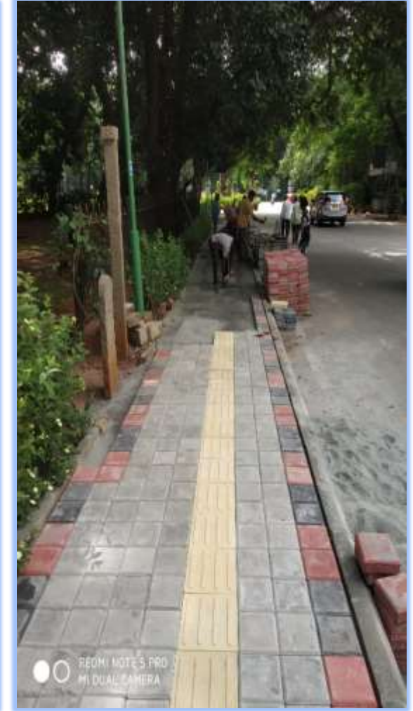
Footpath Improvements, Jogging Track, Laying of Pavers in progress September 2021
